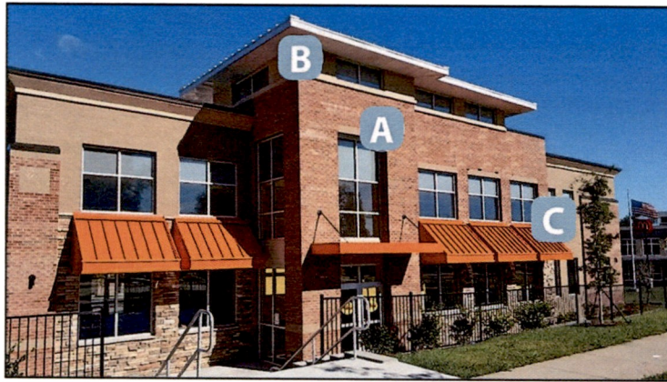
Sample Façade Articulation Elements: Example A.: A=Mid-section windows, B=Clearstory windows, C=Insets, D=Varied rooflines, E=Materials changes
