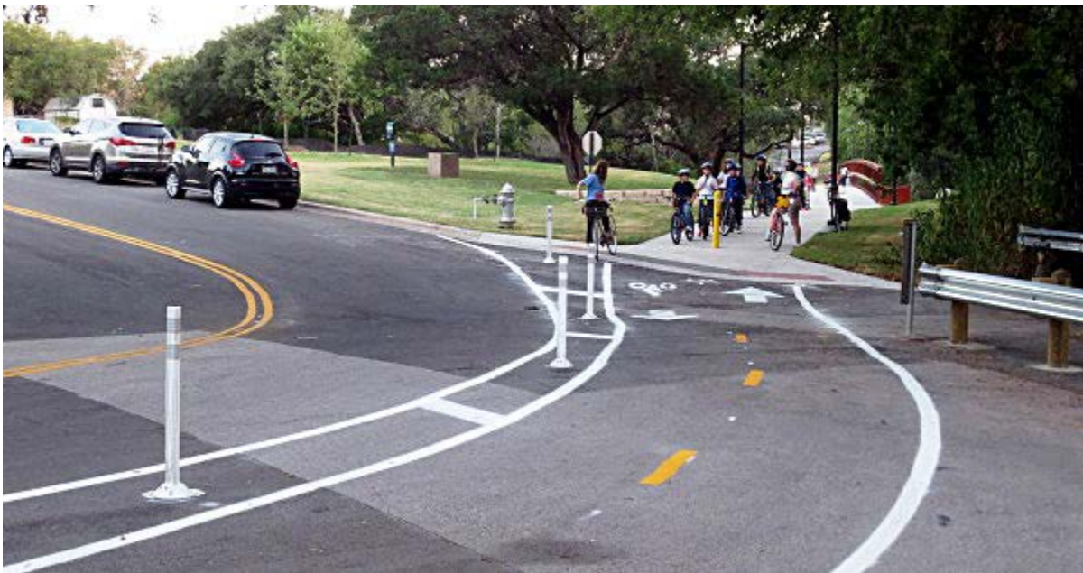
A protected bike lane provides a connection to an existing sidewalk in Austin, TX 88
