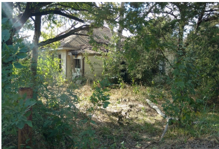
Figure 3C: Example Overgrown Yard/Dilapidated Housing
