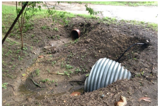
Figure 7B: Undamaged Culvert Example
