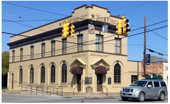
New First National Bank (1902). Style: Colonial Revival
