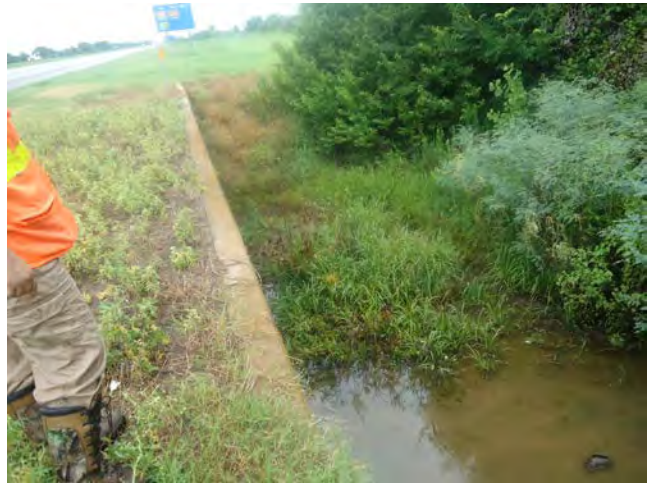
BAUGHMAN SLOUGH BRIDGE CROSSING NEAR NORTH EDGE OF PHASES 3 & 4
