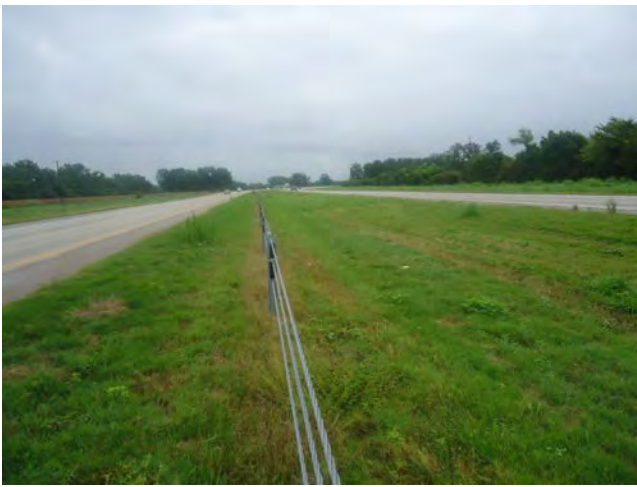
PHASE 4 OVERPASS LOCATION ON HIGHWAY 59 LOOKING SOUTH ALONG MEDIAN
