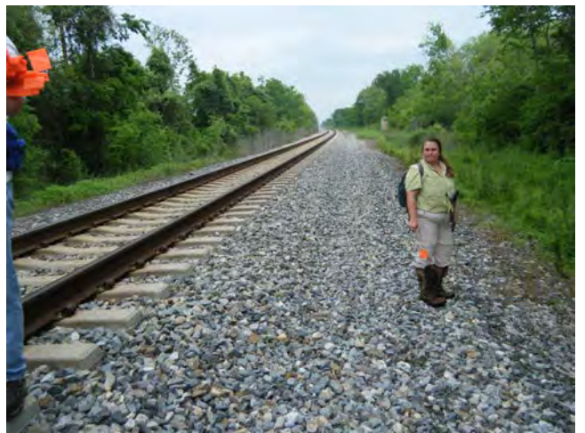
LOOKING NORTH ALONG RR TRACT AT FM 1301 - PROJECT ALIGNMENT
