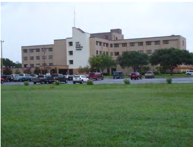
HOSPITAL – EAST OF HIGHWAY 59 NEAR PHASE 3 OF PROJECT
