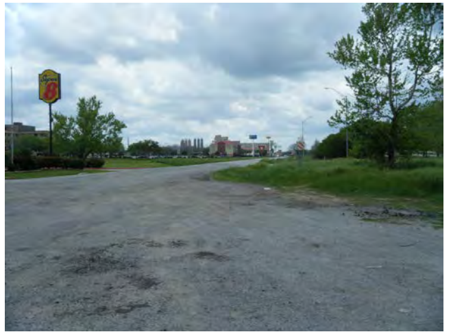
LOOKING SOUTH NEAR SOUTH EDGE OF PROPOSED FEEDER ROADWAY – PHASE 3
