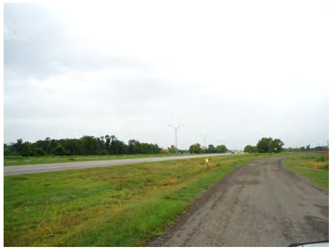
LOOKING SOUTH ALONG WEST EDGE OF HWY 59 PHASE 4 OF PROJECT
