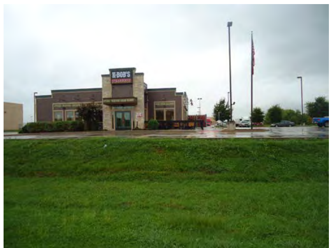
EXISTING COMMERCIAL AREA NEAR PHASE 4 OF PROJECT – SOUTH SECTION
