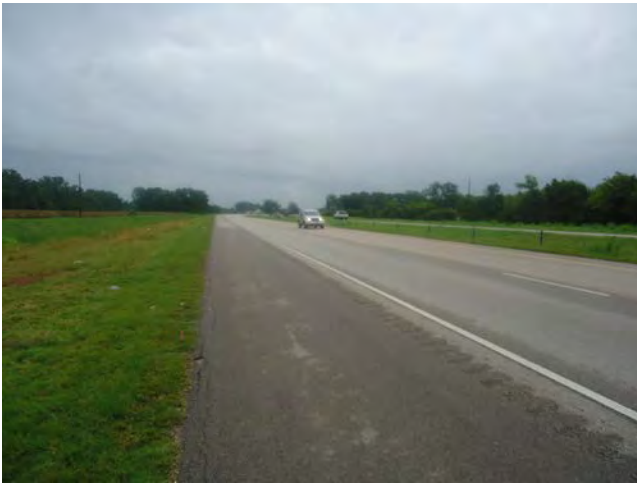
NORTH EDGE OF PHASE 4 LOOKING NORTH NEAR TERMINUS OF PHASES 3 & 4
