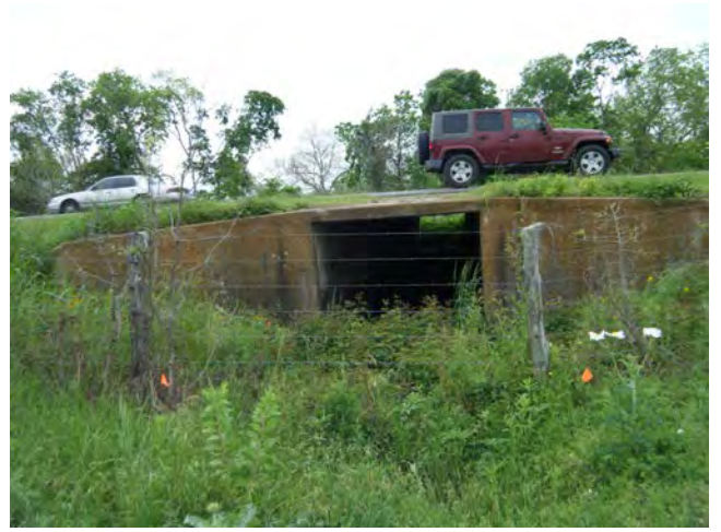
NON WETLAND TRIBUTARY – AT EXISTING BRIDGE FM 102 - PHASE 1 OF PROJECT
